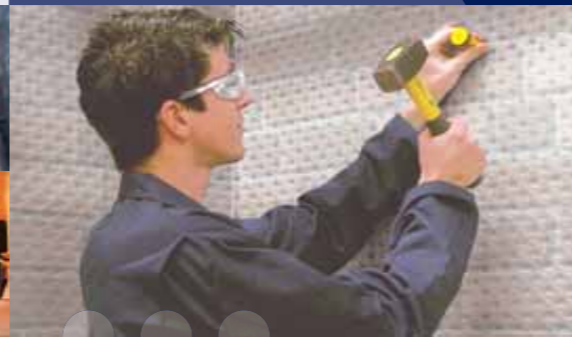
Typical basement waterproofing using Oldroyd Xv clear
