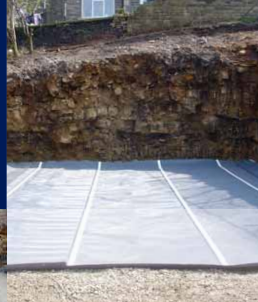
"Double Sealing" detail required when Oldroyd Xs is used as part of a ground gas protection system.
